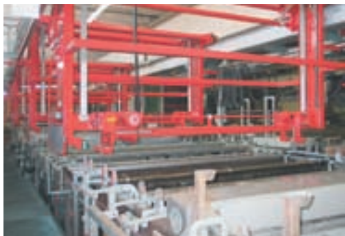
One of the electroplating lines at the Lahr site of Friedrich Grohe
